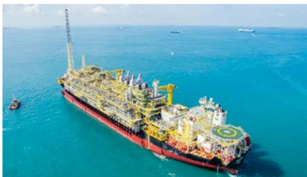
Offshore energy / FPSO (Floating, Production, Storage, and Offloading system) (Brazil)
