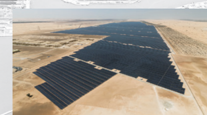
Sweihan Photovoltaic IPP Project
