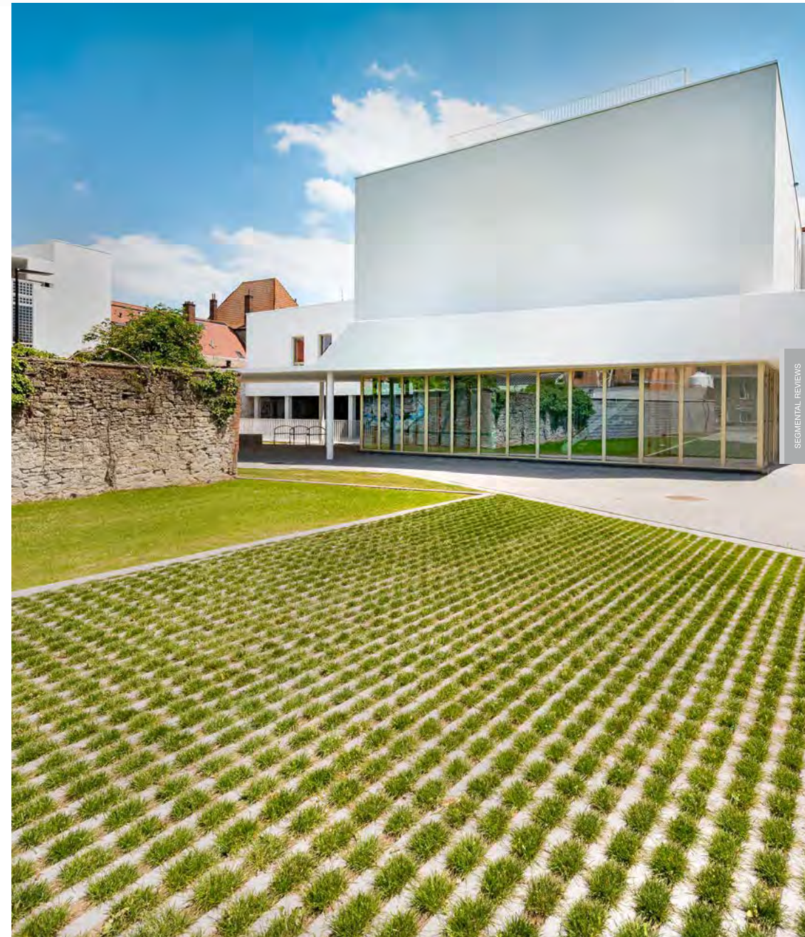
Stradus, part of CRH's Building Products Division, supplied c.1,000 Hydro Lineo XL grass tiles to pave the surroundings of an office complex in Doornik, Belgium. The lattice structure allows water to slowly drain away, keeping the surface free from water while not overloading drainage systems.
