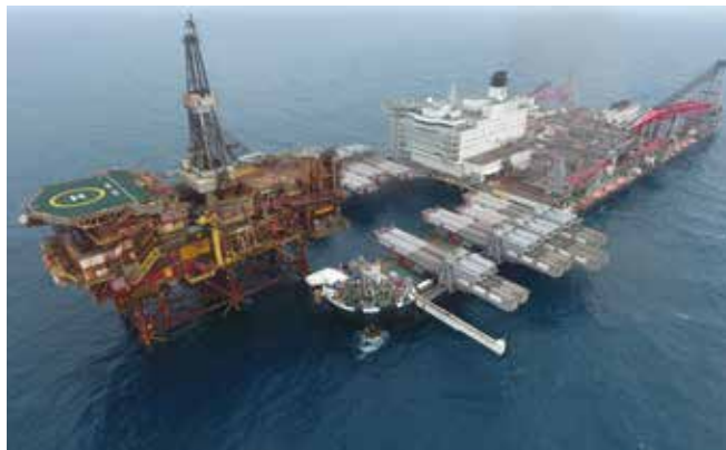
The Pioneering Spirit vessel has now lifted and removed the topsides of Brent Alpha, Brent Bravo and Brent Delta.
