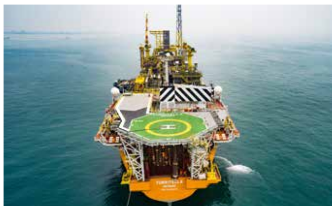
The Turretella FPSO in the Gulf of Mexico.
