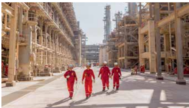
Operators at Pearl GTL plant, Qatar.
