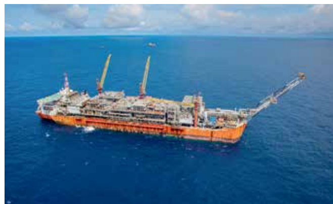
FPSO Bonga, offshore Nigeria.
