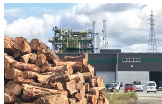
Biomass power generation (Yonezawa, Yamagata Prefecture)
